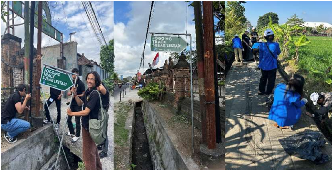
Figure 2. Installation of Direction boards and Jogging Track Arrangement
