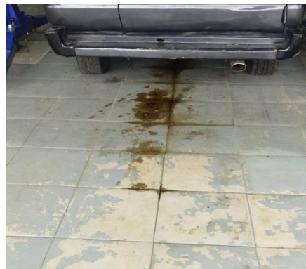
Picture 3 unclean work area
