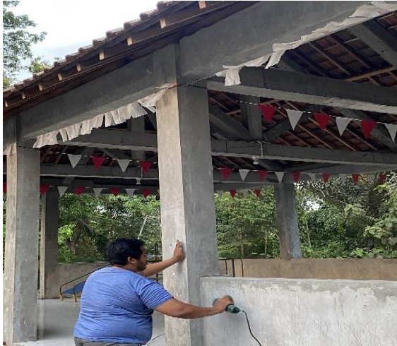
Figure 4. Wall Surface Flattening Process
