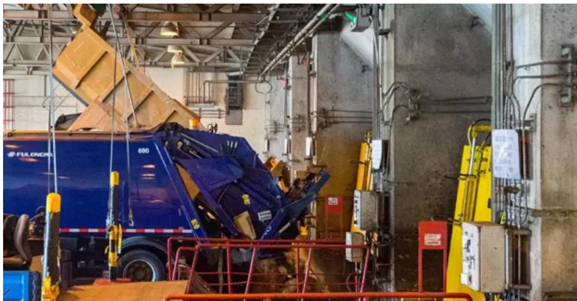
Figure 3. Dump the Trash Into the Pit (Image Source: Government Information Bureau)
