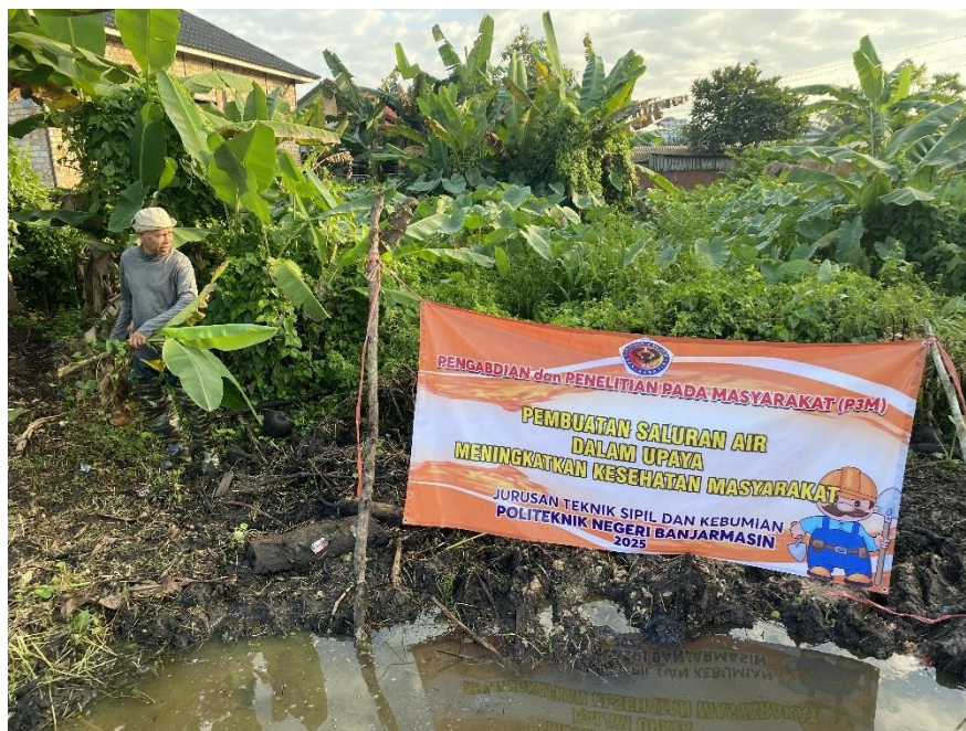
Gambar 2. Proses Land Clearing
