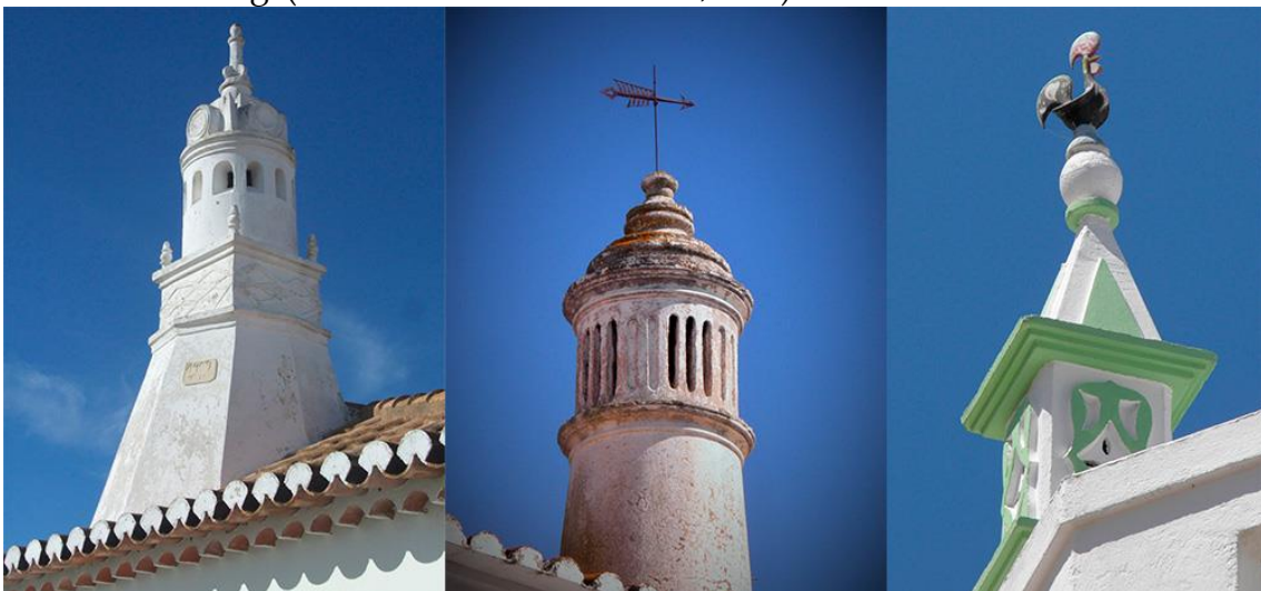
Figure 8. Chimneys (Image Source: Eduardo Moerschbaecher)
