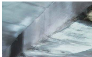
b). Beam surface condition
