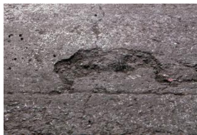
a). Bottom surface Slab condition
