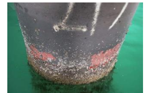
d). Steel pile condition
