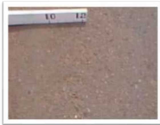
Gambar 16. Pengausan (Polished Aggregate) Sumber: Bina Marga No.03/MN/B/1983
