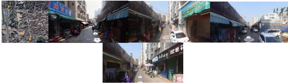
Figure 3-5. The External Area of Wu Gongci, Wu's Great Ancestral Hall and Jie Weng Wu Gongci in Huishan Mountain; Jinhua Temple, Guandi Temple, Caibo Temple; Area A of Road (With The Highest Flow Of People)
