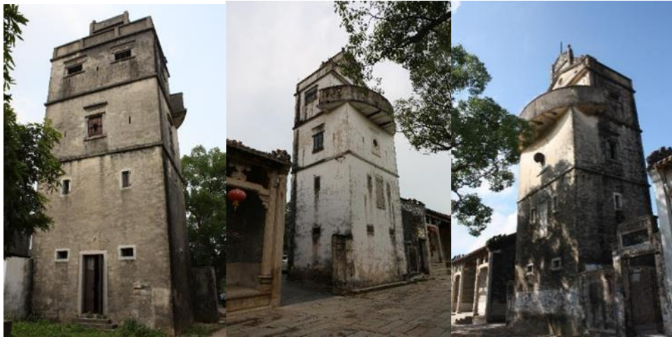
Figure6. Exterior Facade of Huitong South Watchtower
