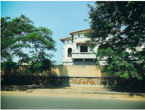
Figure 13. Mansion prepared for demolition Av. Kim Il Sung (Image source: AP1MZ)
