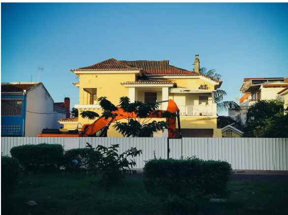
Figure 14. Mansion prepared for demolition Av. Mao Tse Tung (Image source: AP1MZ)
