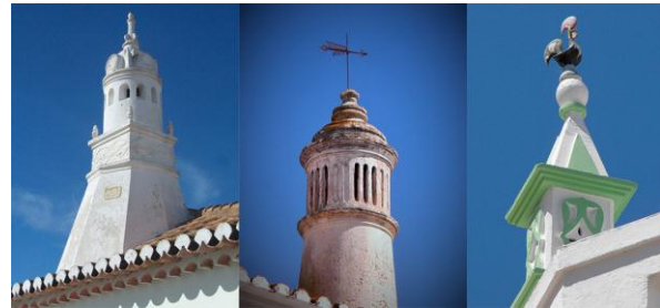
Figure 6. Chimneys (Image source: Eduardo Moerschbaecher)
