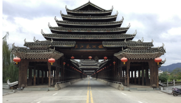
Fig. 6 San Jiang Dong wind and rain Bridge
