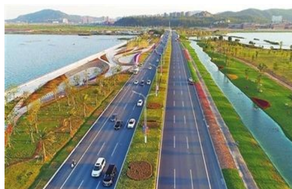
Figure 2. Zhuhai Airport East Road Roadside greening improvement project
