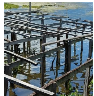
The wooden structure of the anchored house
