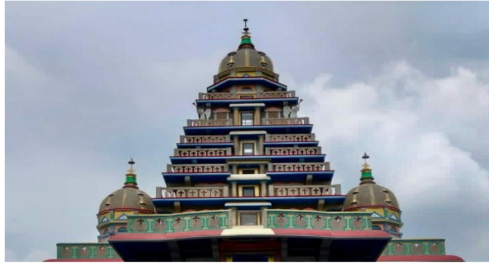
Figure 7. Tower at the Top of the Building
