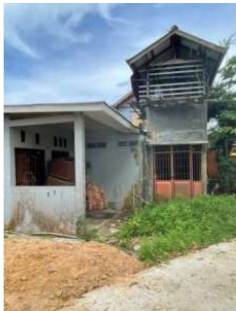
Image 8. The Concrete Structure of the Karang Mumus Source : Author Documentation, 2023
