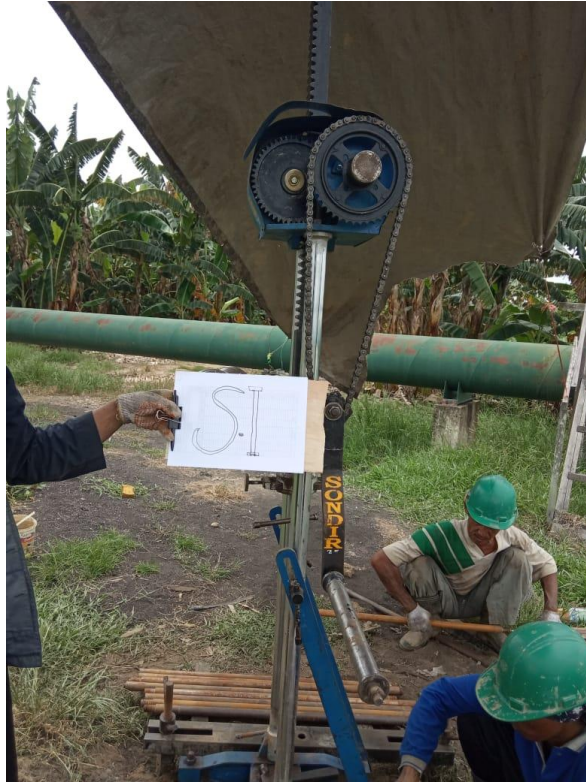
Picture 1. Cone Penetration Test (CPT) Execution at Point 1, Land View
