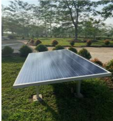
Figure 1. Solar Panel Installation
