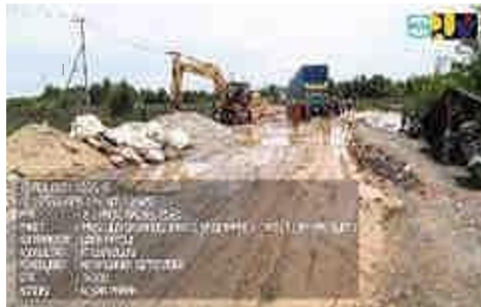
Figure 1. Existing Condition of the Project Site
